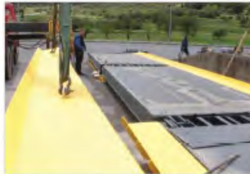
DIY Weighbridge. Installation of side rails
