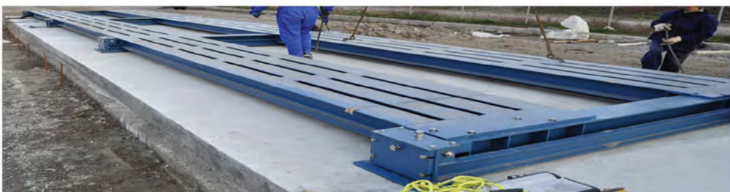
TS-300 weighbridge. Installation
