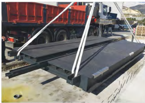
NT31-3 weighbridge. Easy installation
