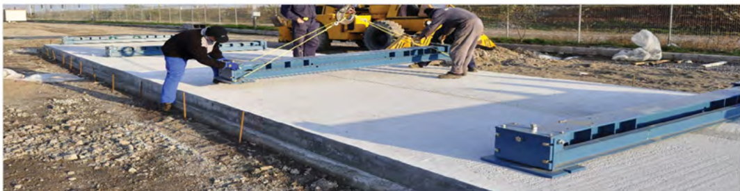
TS-300 weighbridge. Weigh modules placement /installation
