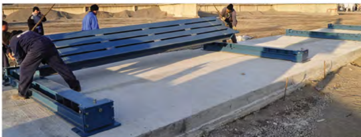
TS-300 weighbridge. Weigh modules placement /installation
