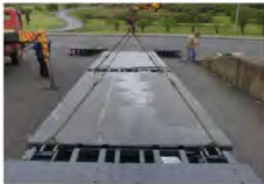
DIY Weighbridge. Installation of main body
